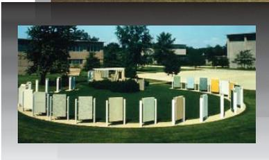
*Figures. In 1962, newly erected panels at PCA's property near Chicago put bright new faces on concrete surfaces. The display consisted of a circular walkway in exposed aggregate concrete, and white cement concrete posts supporting two panels placed back-to-back. [IMG14306, IMG15614]*
