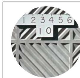
**Panel 10:** This panel is a forerunner of today's wide array of formliners. Sharp edges were softened over the years by minor paste erosion. (IMG14238)
