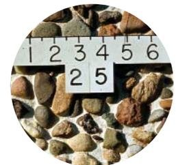
**Panel 25:** This panel was vertically cast by first consolidating aggregate in forms coated with surface retarders, then removing the forms, washing and brushing away surface paste, and sandblasting to deepen the texture. (IMG13754)
